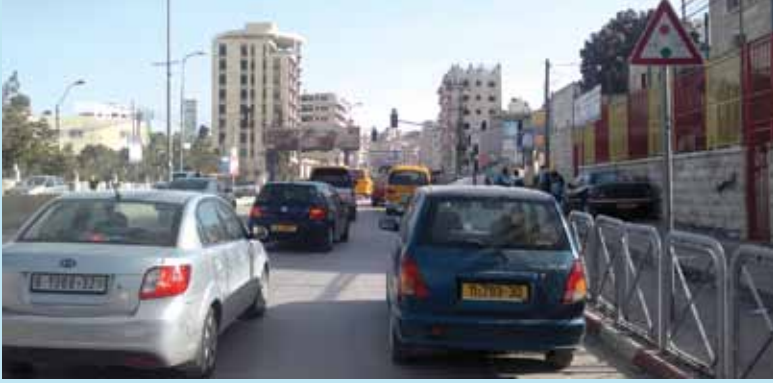
Faulty traffic lights at Samiramees junction between Ramallah and Jerusalem. Photo courtesy of PECDAR.
